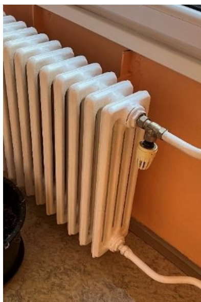
Obr. Detail OT s TRV
