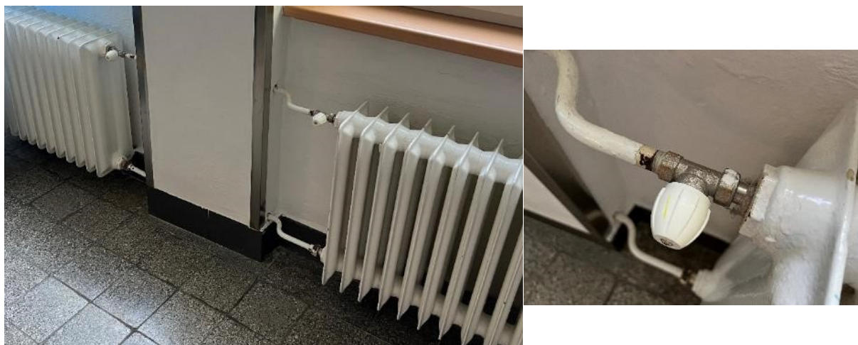
Obr. Detail OT a ventilu
