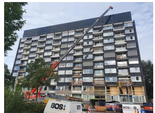
Figure 1.8 The first retrofitted high-rise Positive Energy Building in Europe completed in Overvecht-Noord Utrecht in 2020.
