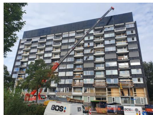
Figure 1.8 The first retrofitted high-rise Positive Energy Building in Europe completed in Overvecht-Noord Utrecht in 2020.
